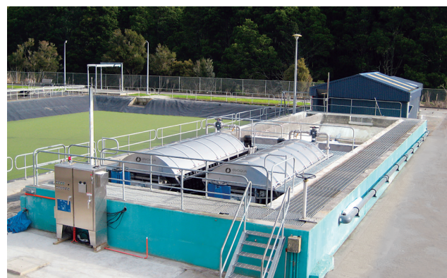
The Forty-X™ Disc Filter requires a fraction of the footprint required by traditional sand filters increasing capacity and performance
